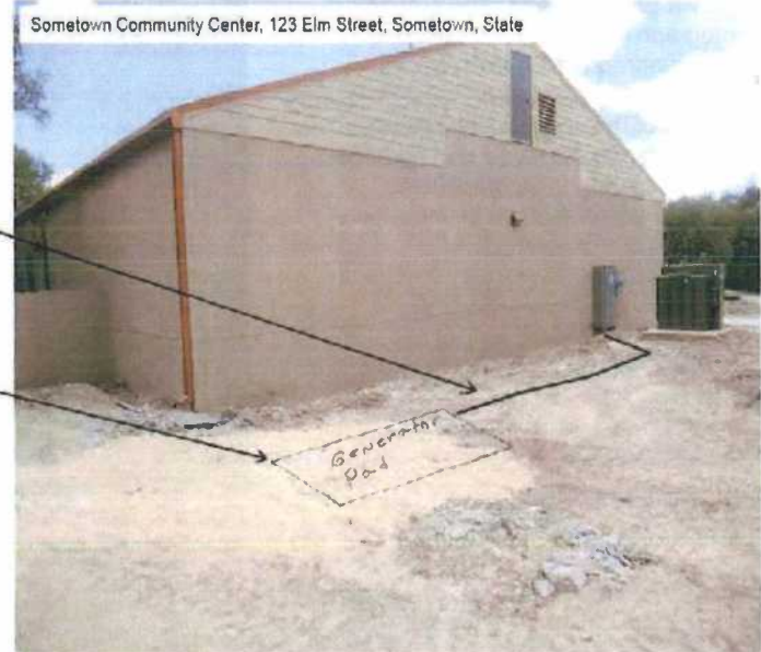
Figure 4. Ground-level photograph showing proposed ground disturbance area.
