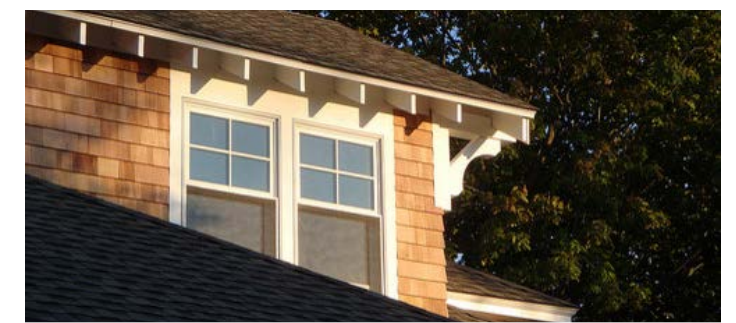
EXPOSED BEAMS/RAFTER TAILS
