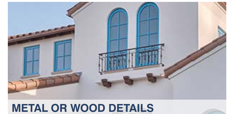
METAL OR WOOD DETAILS These can be used for staircases, balconies, railings, or other decorative elements like gates and window guards. Metal can be wrought iron, bronze, or black painted tubular steel.
