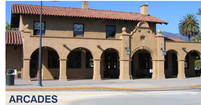
ARCADES Use of arcaded walkways (row of arches supported by columns or piers)
