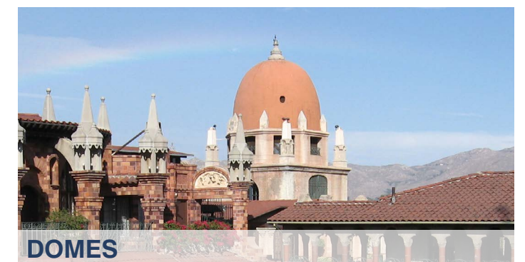
DOMES A rounded vault forming the roof of a structure, typically with a circular base
